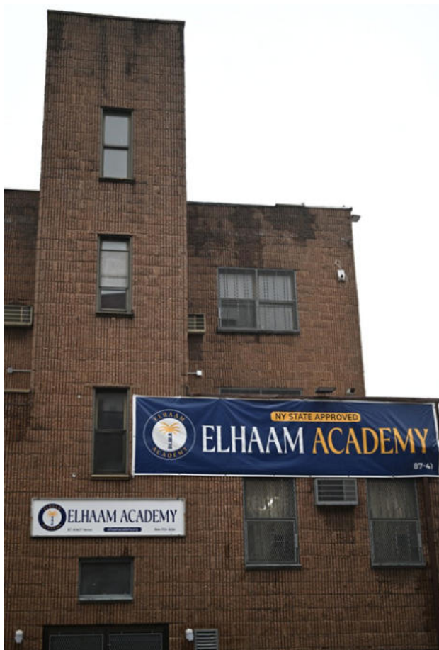
Photo: Elhaam Academy at 87-41 165th St.
