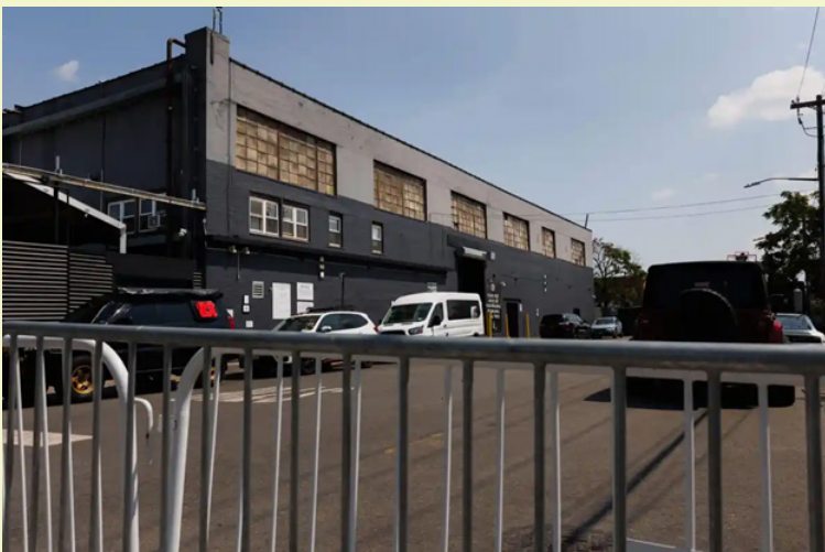
Photo: The Brooklyn Mirage is set to be demolished starting next month
